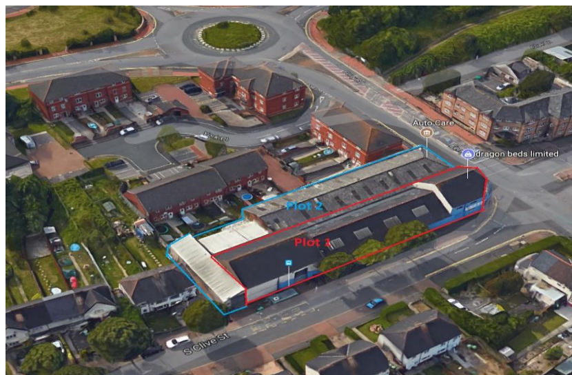
aerial view of site
